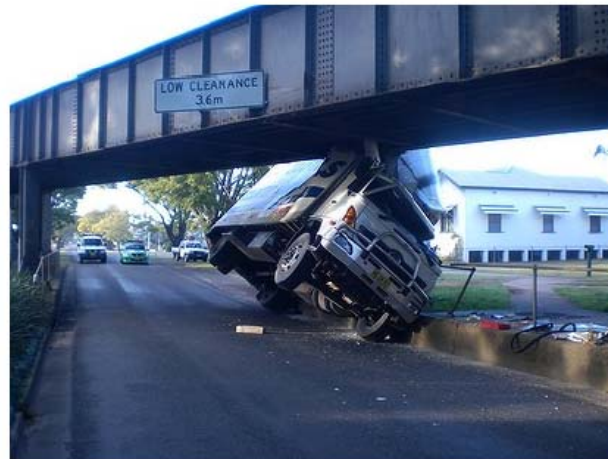
Well and truly stuck ... the truck under the bridge at Grafton. Photo: Daryl Halliday Sydney Morning Herald: July 22, 2009
